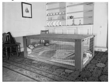
designed to protect occupants from masonry and debris if the house was hit by a bomb.
